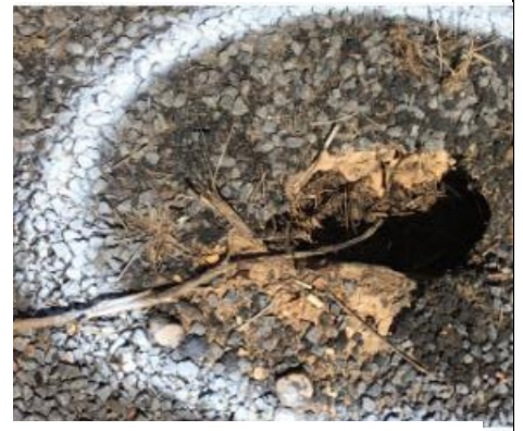
Close up, angled views of marked up undermined site.
