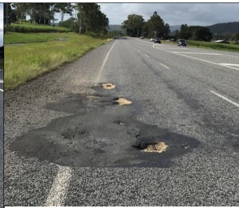
Above – geotagged photo examples of post event pothole damage requiring emergency patching
