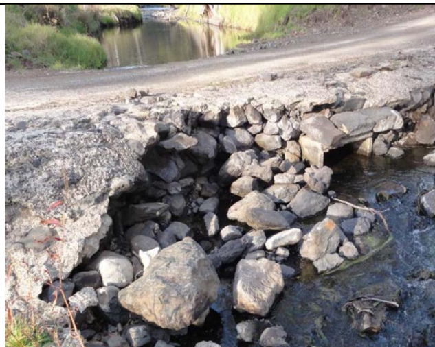
Undermined floodway
