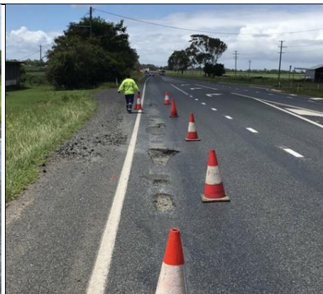
Above – geotagged photo examples of post event pothole damage requiring emergency patching
