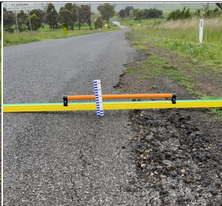
Series of four photos utilising asset mark up, straight edge and measures to support extent of damage at the site, depth, width and length
