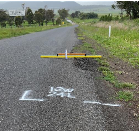
Series of four photos utilising asset mark up, straight edge and measures to support extent of damage at the site, depth, width and length
