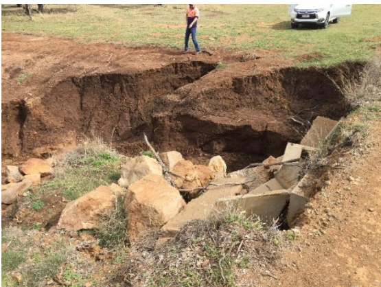
7. Photo further demonstrating extent and scale of event damage at site.
