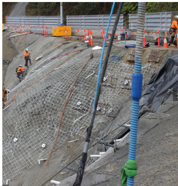
Scope of works in progress
