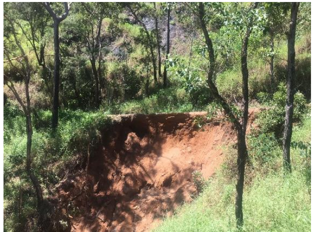
View back at slip and asset
