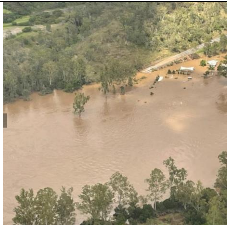
Post event drone view of road crossing
