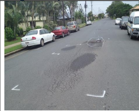
Mark up showing dimensions of event damage and proposed scope.
