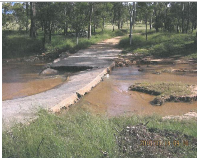
Undermined floodway
