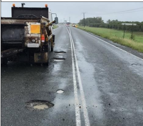
Above – geotagged photo examples of post event pothole damage requiring emergency patching
