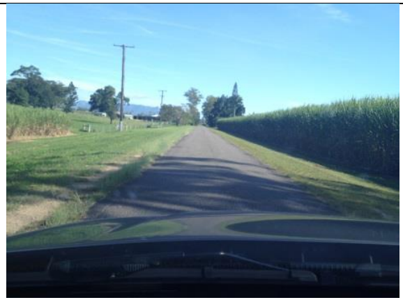
Photos taken through windcreens, and dark shadows across asset do not show extent of event related damage to the asset
