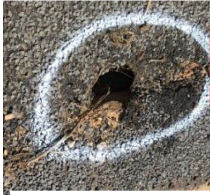
Close up, angled views of marked up undermined site.
