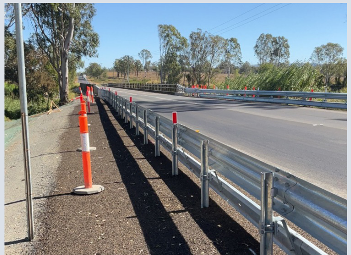
Lockyer Creek Bridge – restored guardrail prior to final line-marking (March 2023)
