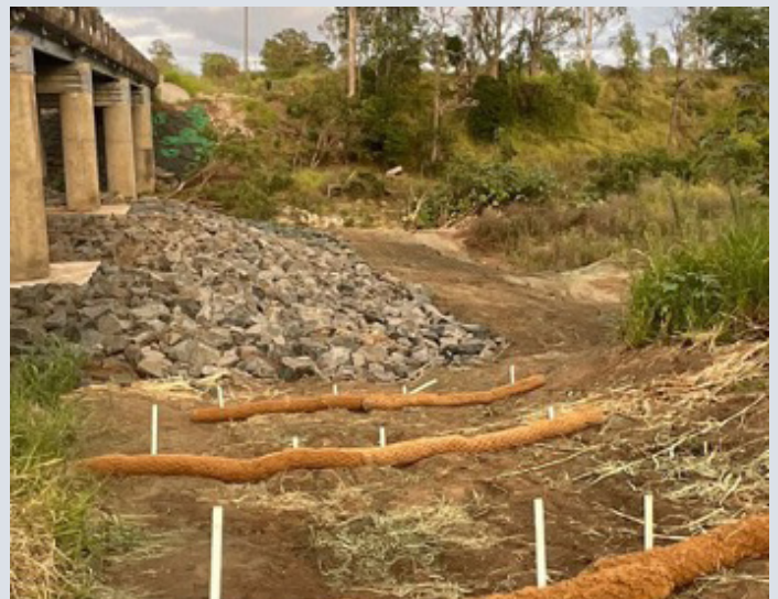
Lockyer Creek Bridge – restored rock protection (January 2023)
