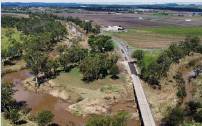
Gatton–Helidon Road – emergency works in progress at Lockyer Creek Bridge (March 2022)
