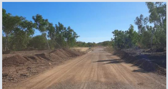
Gregory Downs–Camooweal Road – emergency works to remove gravel from road (June 2023)
