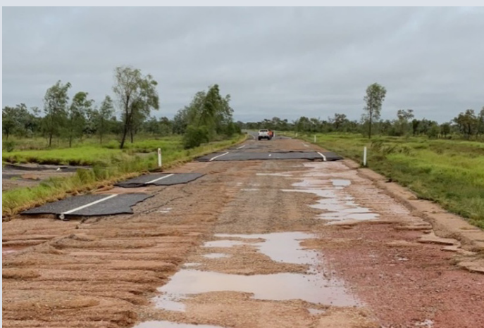
Barkly Highway (Mount Isa–Camooweal) at Nowrairie Creek – damage from Northern and Central Queensland Monsoon and Flooding (March 2023)
