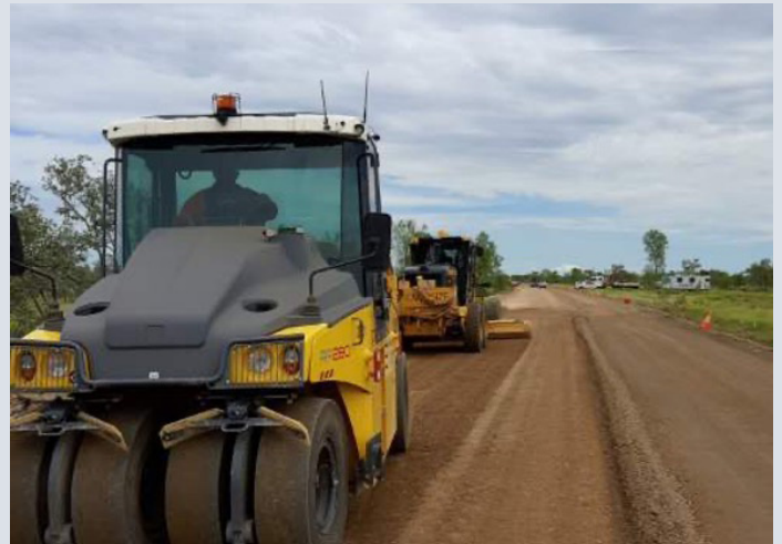
Barkly Highway (Mount Isa–Camooweal) at Nowrairie Creek – emergency works (March 2023)
