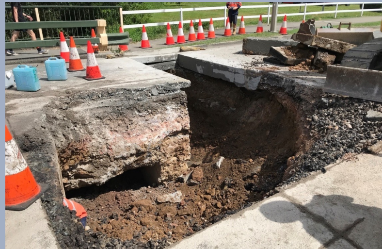
Image: Gympie Arterial Road – loose materials being excavated.
