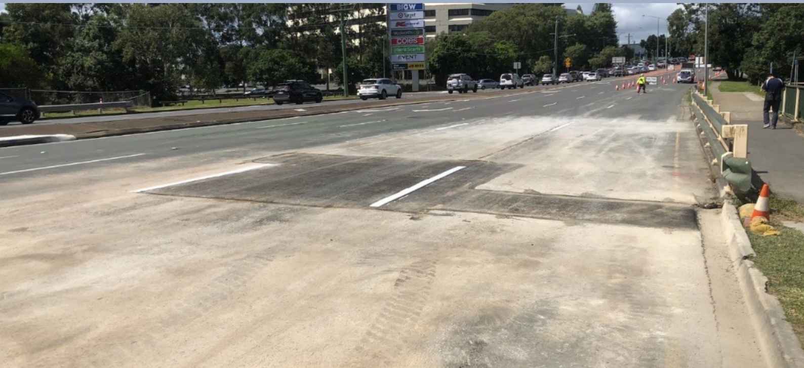
Image: Gympie Arterial Road – completed emergency works.
