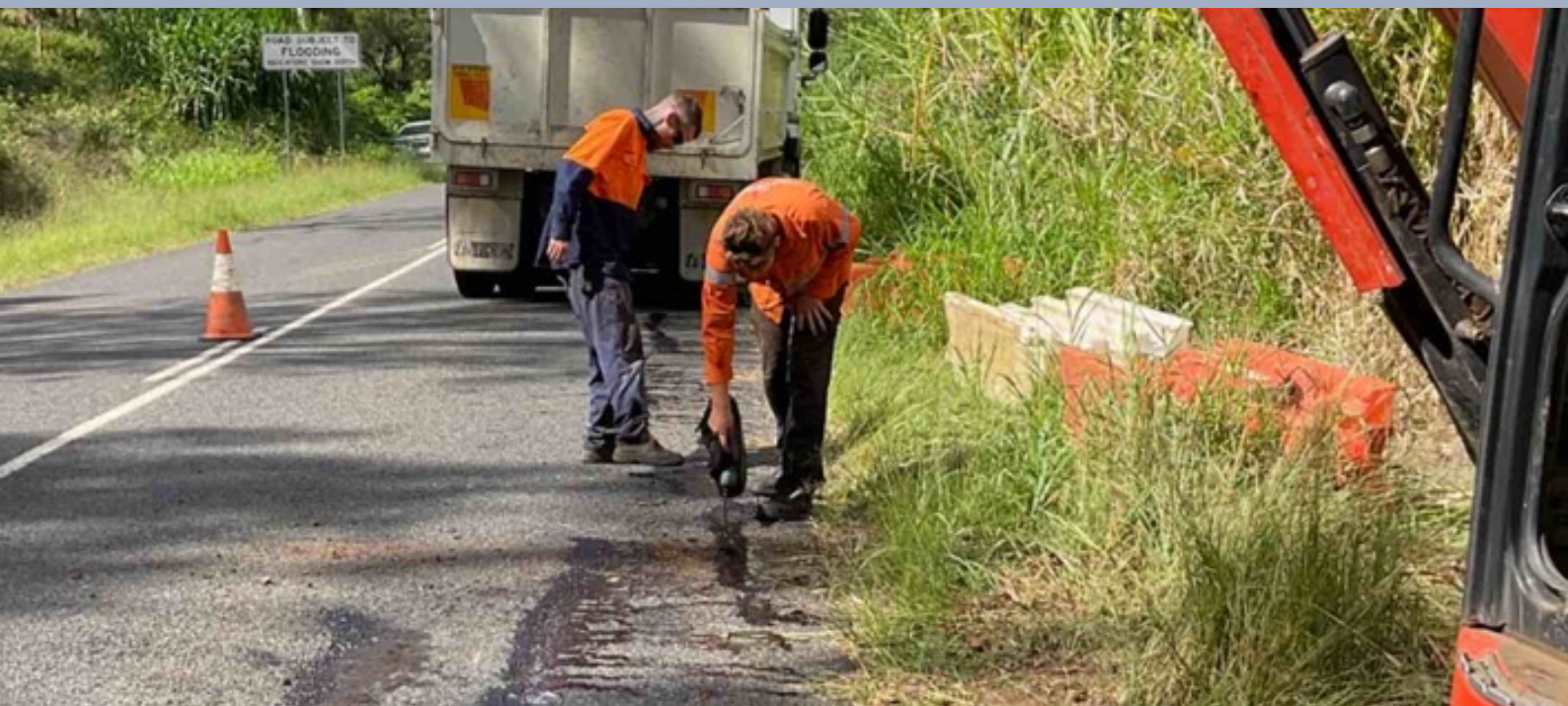
Image: Mulgowie Road – road crew repairing cracks with sealant (March 2022).
