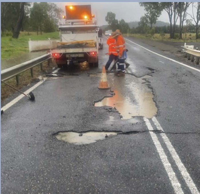
Image: Bruce Highway (Gin Gin–Benaraby). Emergency works
