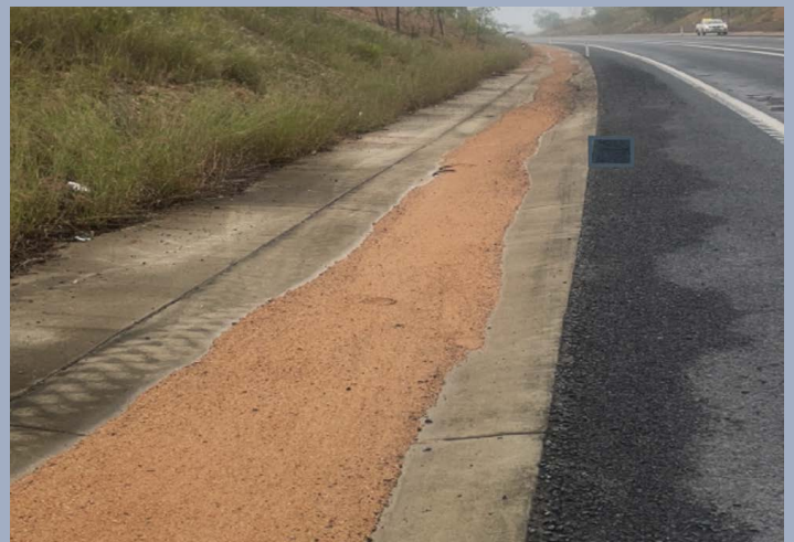
Image: Bruce Highway (Gin Gin–Benaraby). Silt build-up on road shoulder at Cabbage Tree Creek.
